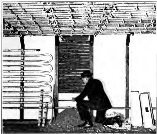
Panel system of cork insulation showing panel removed for inspection.
